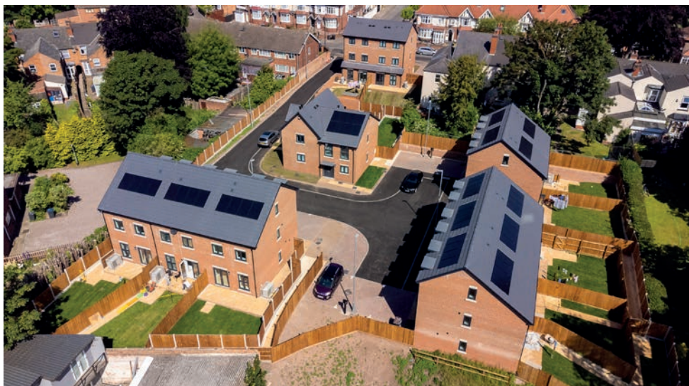
Figure 2: Midland Heart Project 80. A 12 homes demonstrator built to the Future Homes Standard
